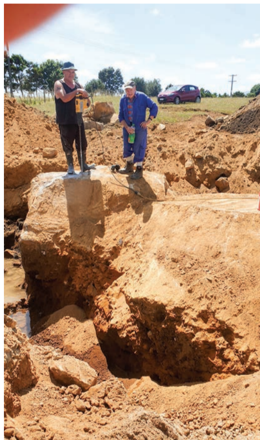
All in a day's work for Len Pentelow.
